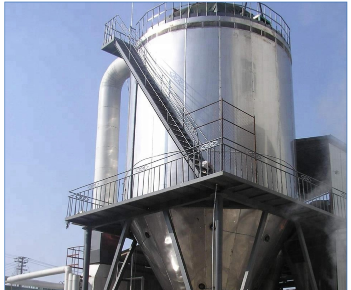
Industrial Spray Dryer
